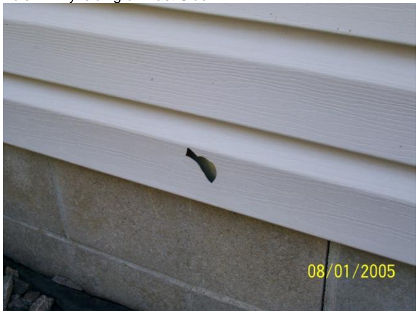
Hole in vinyl siding on East Side
