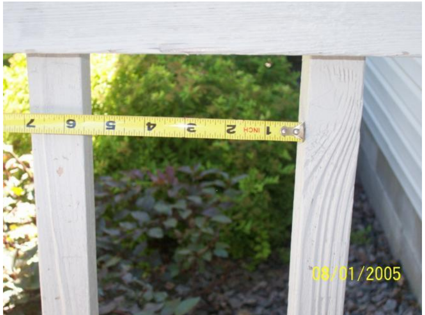
Railing balusters spaced to far apart, No more than 4" max. recommended
